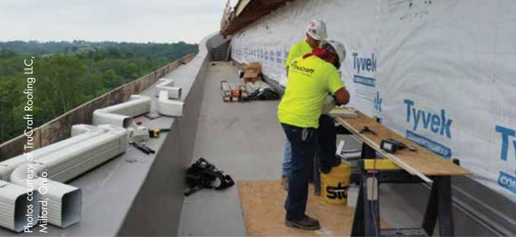
From left to right: TruCraft Roofing workers install the ark's gutters and edge metal; workers adhered TPO membrane in slate gray
